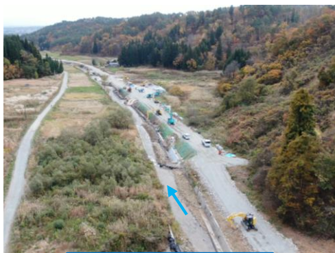
萩生川(飯豊町萩生地内)護岸復旧
