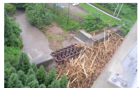
写-8 流木捕捉の事例(透過型砂防えん堤)
